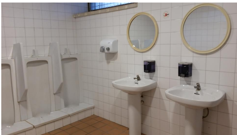
SERVEIS GENERALS. BANY HOMES
